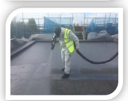
UKG recommended the full overlay of existing roof with a New 120mm Warm Roof Overlay System, using Prokol 260 FR Pure Polyurea Hotspray roof coating.
