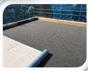
On request of the client UKG surveyed the roof areas for new external works applications. Core sampling was carried out with reports submitted to Kingspan for Insulation specification to BBA Certification. There were three number flat roof areas with an aluminium capped brick parapet wall.
